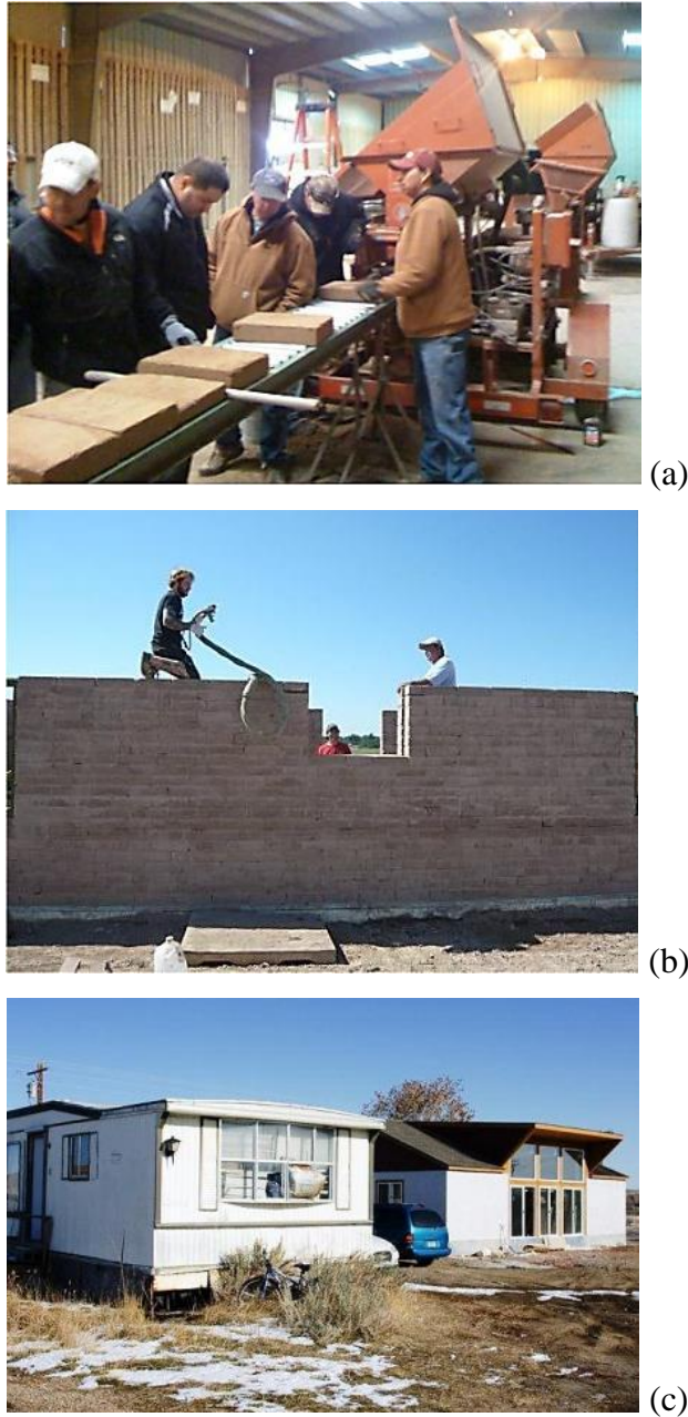
Figure 1.1 Crow Tribe's Good Earth Lodges operation: (a) block fabrication in local facility, MT; (b) construction; and (c) finished dwelling structure (right) replacing nearby trailer home (left). Credit: Thomas Bowen (a-b) and Patrick Bresnan (c).
