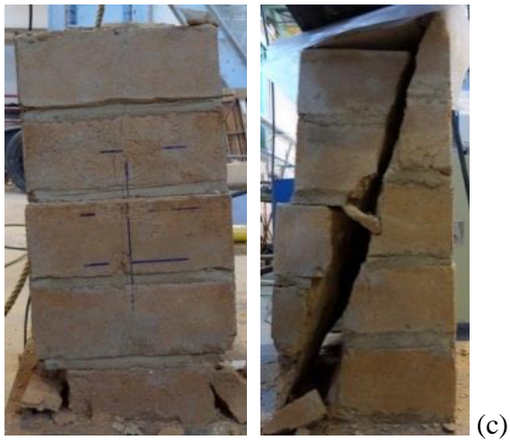
Figure 3.11 Representative failure mode of masonry prisms: (a) C, (b) CS6, and (c) CS9 specimens.
